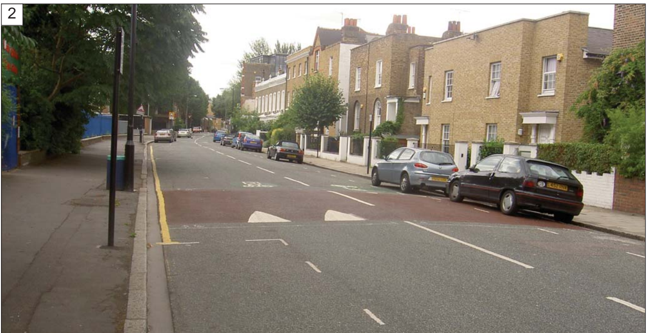
Scheme Photo: 2 Scheme Reference: BS\05\LCN\LAM.04 Location: Larkhall Lane (between Priory Grove & Lansdowne Way) Link number: 129 Description: Implementation complete for traffic calming on Larkhall Lane and junction improvements at Larkhall Lane/Lansdowne Way. Design completed for improvements to cycle point no entry at Priory Grove. Length: 0.32km Cost: £64,512
