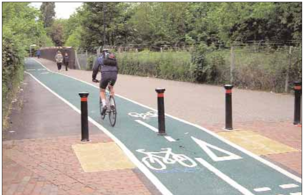
Above: Eddystone Bridge segregated cycle path. Below: Brookmill Park
