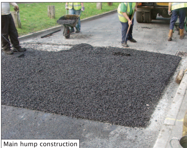
Inner section of the hump being laid
